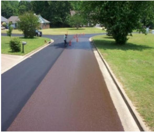
Figure 44 - Good Surface Texture Uniformity
