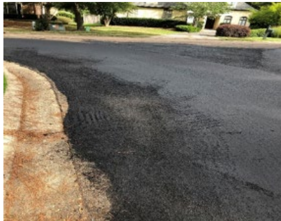
Figure 70 - Unacceptable Handwork
