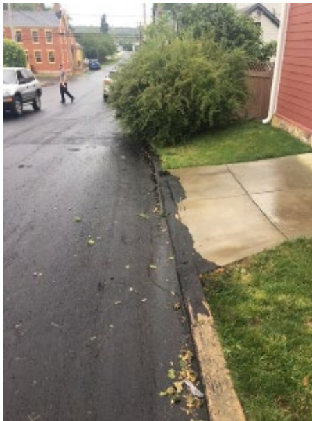
Figure 61 - Mix on Curb/Driveway
