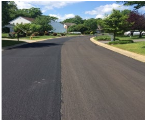
Figure 49 - Non-Uniform Color after Curing
