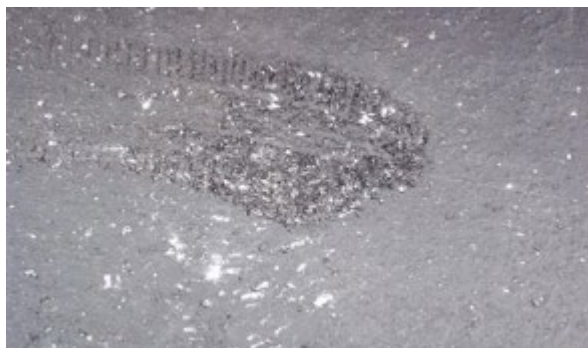
Figure 47 - Minor Surface Scuffing/Power Steering Marks
