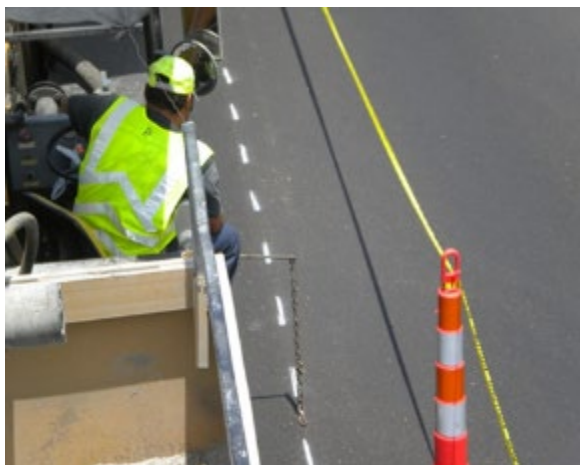
Figure 43 - Use of Pilot Line
