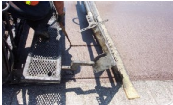
Figure 30 - Creation and Repair of a Drag Mark
