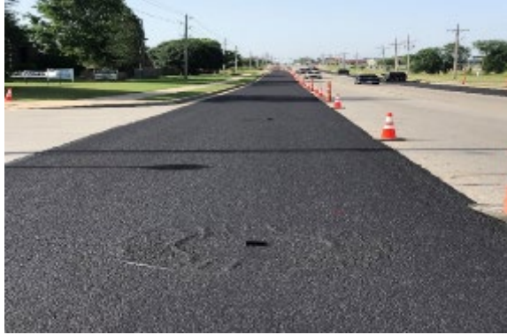
Figure 12 - Flexible, Temporary Chip Seal Marker and Properly Utility Masking (after application)
