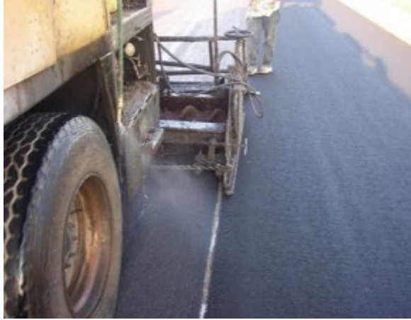
Figure 37 - Construction of a Good Longitudinal Joint
