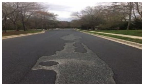
Figure 57 - Delamination
