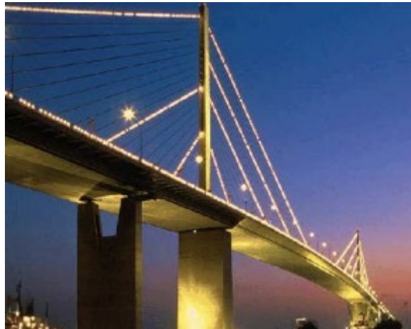
Figure 2 - Ralumac Micro Surfacing – King Rama IX Bridge, Bangkok
