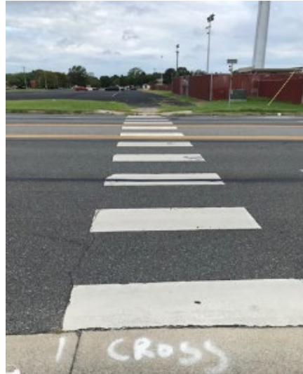
Figure 72 - Existing Thermoplastic Markings
