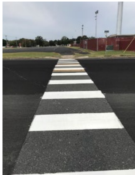
Figure 73 - Protecting Existing Thermoplastic Marking Prior to Micro Surfacing (at customer's request – not recommended as ridges will create ponding of rainwater)
