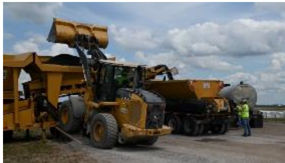
Figure 6 - Typical Aggregate Stockpile
