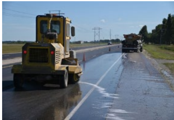
Figure 9 - Surface Cleaning to Remove Tracked Dirt and Mud
