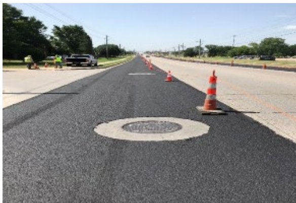
Figure 13 - Removal of Masking Following Proper Curing of Slurry Surfacing
