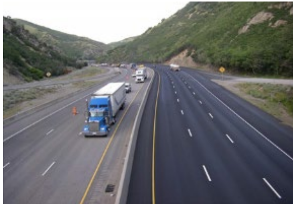
Figure 1 - Slurry Surfacing System Project
