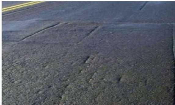
Figure 28 - Excessive Drag Marks Created by Poor Spreader Box Maintenance
