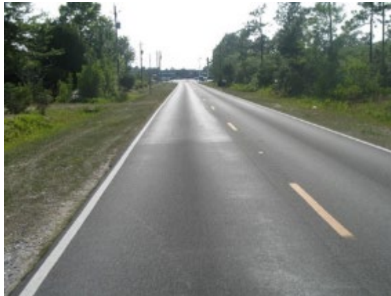
Figure 51 - Flushing
