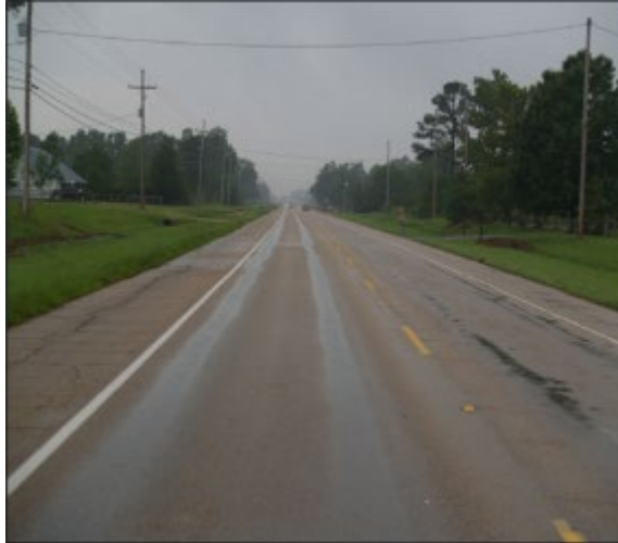
Figure 25 - Acceptable Candidate for Rut Filling
