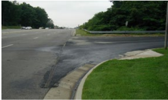
Figure 36 - Poor Mixture Consistency – Excess Total Liquids
