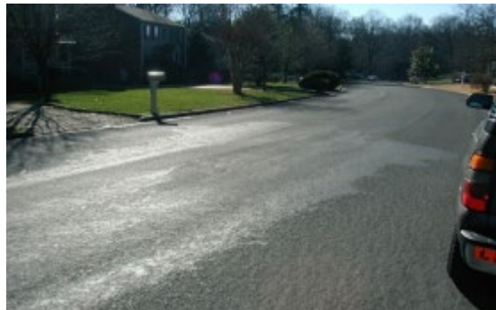
Figure 53 - Lack of Uniformity at the Beginning/End of Passes
