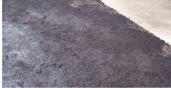
Figure 54 - Unsatisfactory Handwork
