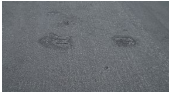
Figure 55 - Power Steering Marks
