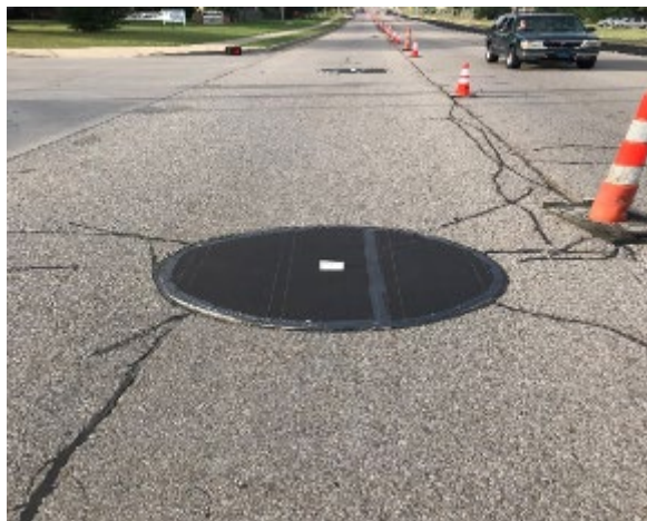
Figure 11 - Flexible, Temporary Chip Seal Marker and Properly Utility Masking
