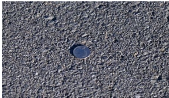
Figure 34 - Fine Surface Texture
