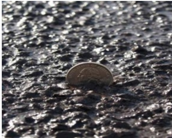
Figure 45 - Magnified View of High Friction Surface Texture
