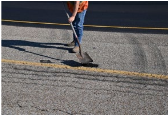
Figure 16 - Repairing Hole (from previous picture) with High Performance Cold Mix
