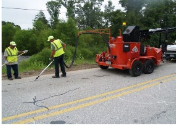
Figure 8 - Crack Treatment Prior to Application
