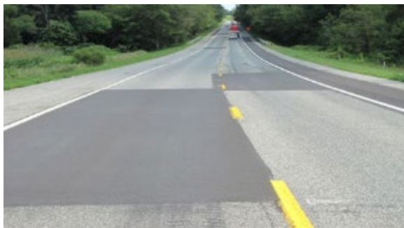
Figure 7 - Proper Pre-Application Patchwork
