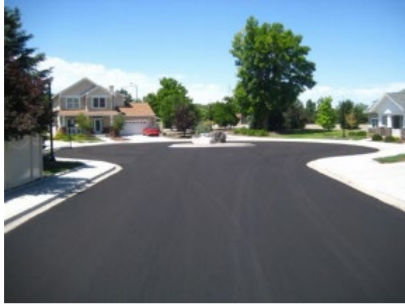
Figure 71 - Finished Treatment on Cul-de-sac
