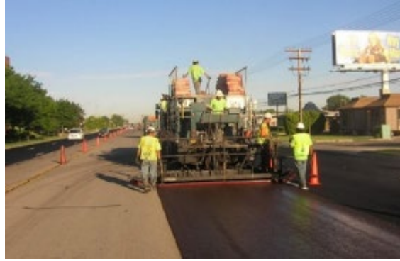
Figure 3 - Application of a Slurry Surfacing System Treatment
